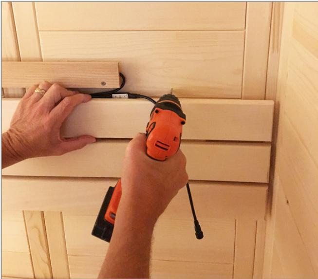
**STEP 3** - Locate where you want the cord to exit the sauna. Drill a 5/8" hole through the sauna wall
