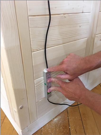
**STEP 6** - Mount the power supply to the exterior sauna wall, ceiling or other place where you can secure with either screws or small nails (not included). Plug the power supply into a 110v outlet and turn on the On/Off LED switch.
