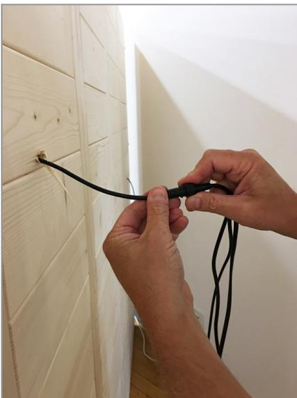
**STEP 5** - On the exterior of the sauna connect the power supply to the LED bar cord. NOTE: Be sure the connection is secure and the nut is firmly hand-tightened.
